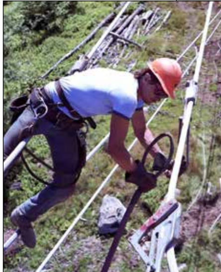
Joe in action wearing his Bashlin 88 belt with homemade rope safety.
