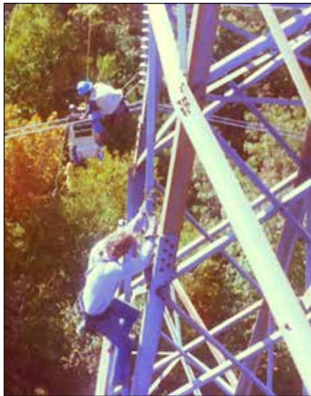
Joe in action wearing his Bashlin 88 belt with homemade rope safety.
